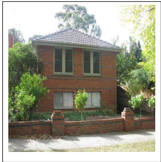
Picture of the front of the new "Lions House" interim facility
