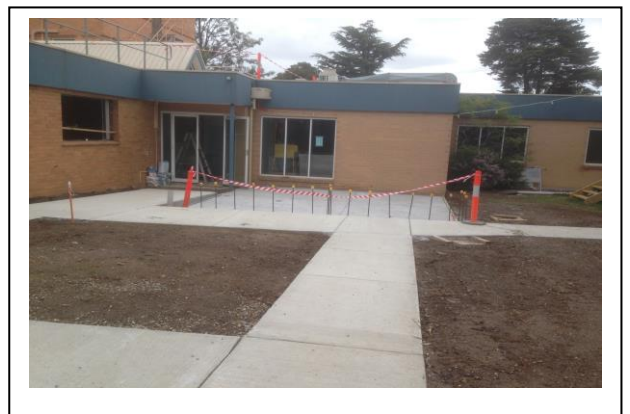
External view looking to front entrance and outdoor paved area
