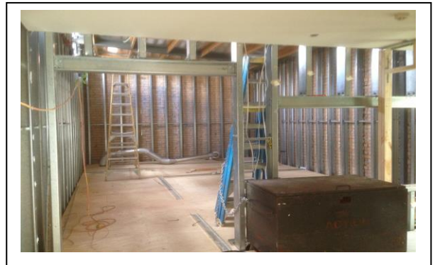
Internal photo of new bedroom area
